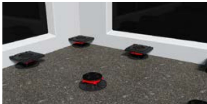
Place the pedestals on the ground, spacing them according to the size of the slabs
