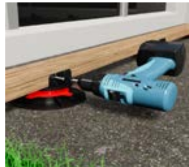
Screw the joists onto the pedestals, through the lugs
